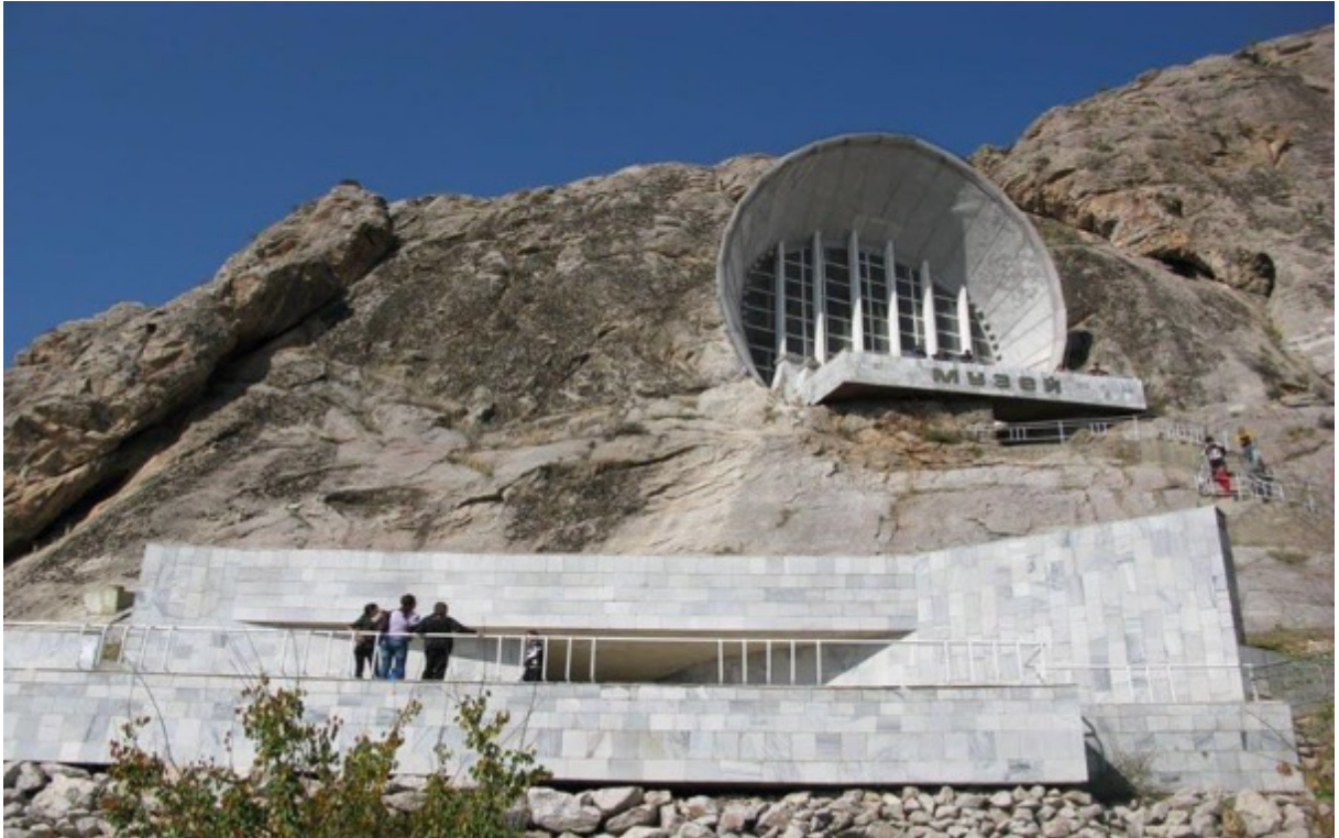
Figure 12. Front View of Lower & Upper Podium
