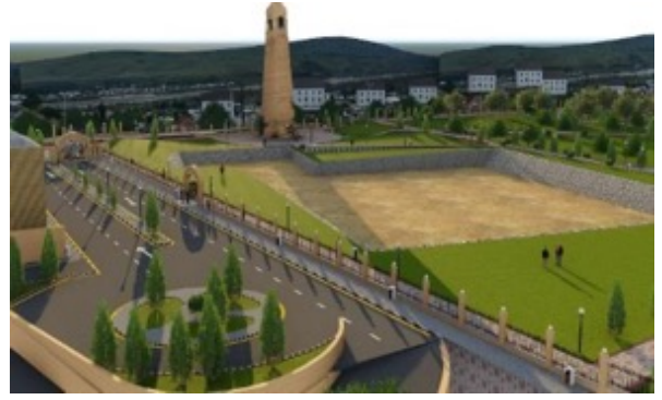
UHAC territory modernization project
